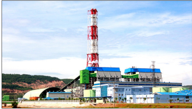
Nghi Son 1 Coal-fired Thermal Power Plant
