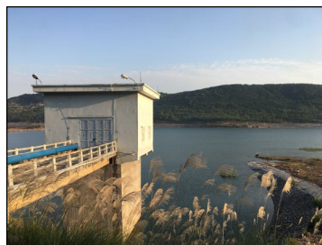
Ash Disposal Pond
