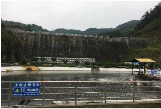
Leachate treatment facility (Guizhou Province) (photo : Ex-Post Evaluation Report)
