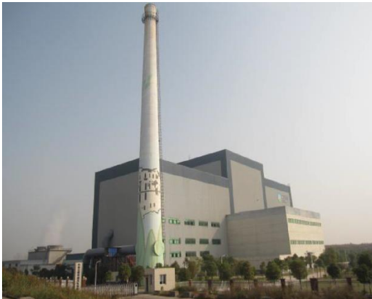
The household waste incineration facility that was built (Anhui Province) (photo: Ex-Post Evaluation Report)
