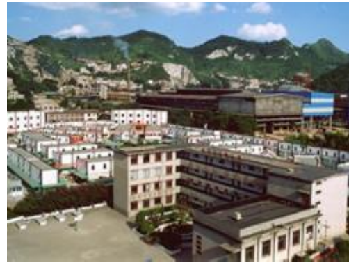
Same steel plant after the project (photo: Ex-Post Evaluation Report)
