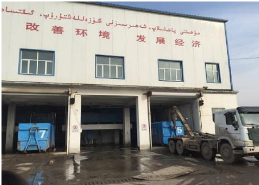
Transfer station (Xinjiang Uygur Autonomous Region) (photo : Ex-Post Evaluation Report)
