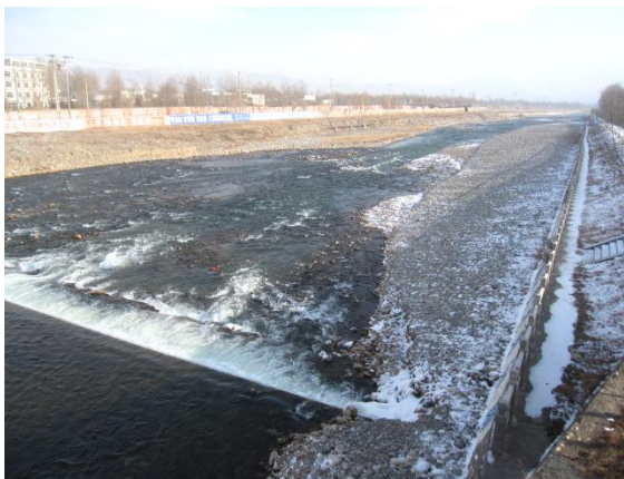
Revetment protection work under the Project
