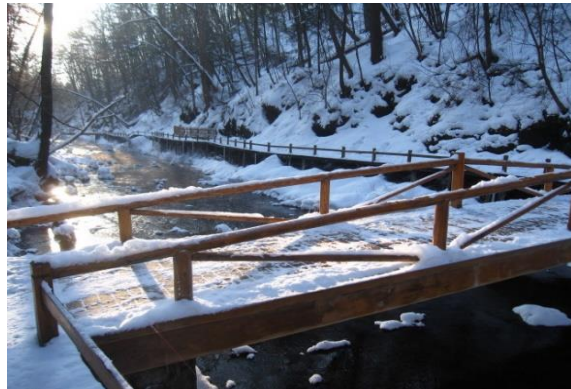
A footpath built under the Project (Model forest ecology park)
