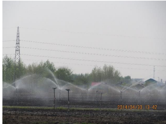
Sprinkler system introduced under the Project
