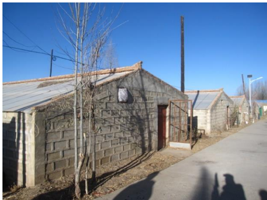
Animal shed constructed under the Project
