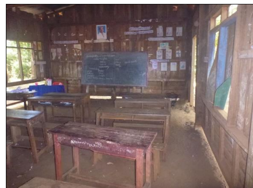
Temporary school building (not constructed by this project)
