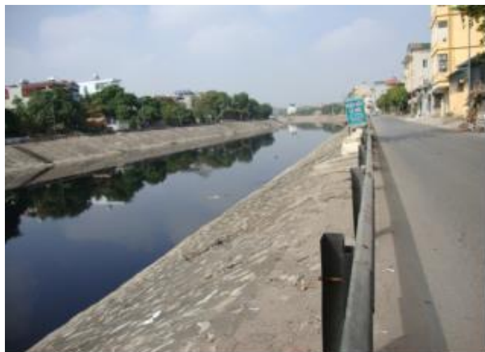
An upgraded canal and road
