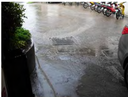
Drains through existing drainage system (Inlet Manhole in a parking area).
