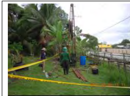
Relay Tank-2: Highest point in the transmission pipeline
