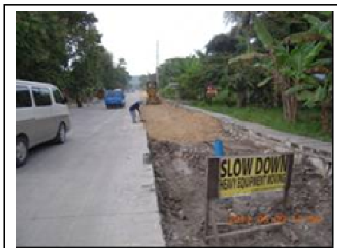
Center Highway in Panglao Island under expansion work
