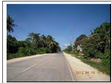
Center Highway in Panglao Island before expansion work
