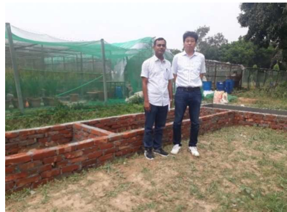
Image 3: Monitoring the structure by Prof. Hoque and Mr. Kasatani
