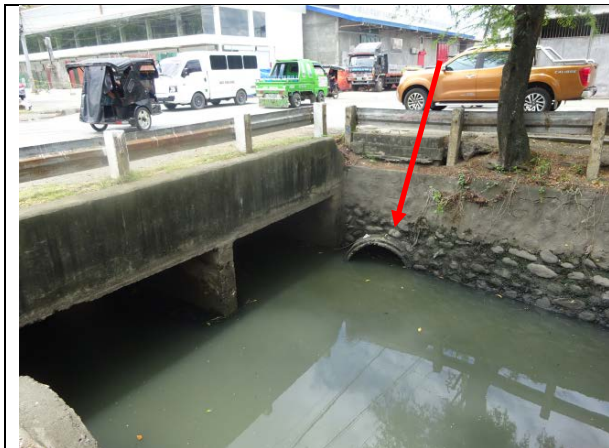
Photo 6.3.4 Submerged Outfall in Dacudao Creek
