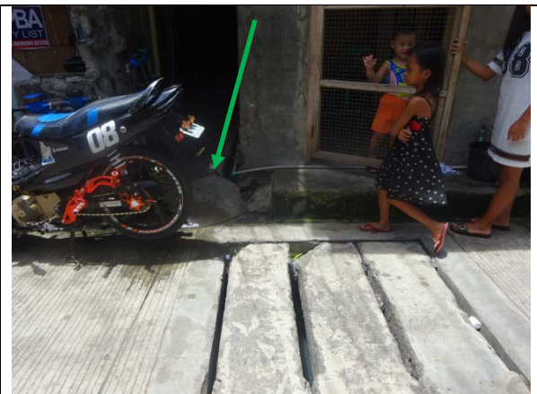
Photo 6.3.3 One Exit of Wastewater from a Congested area in Barangay Tomas Monte Verde
