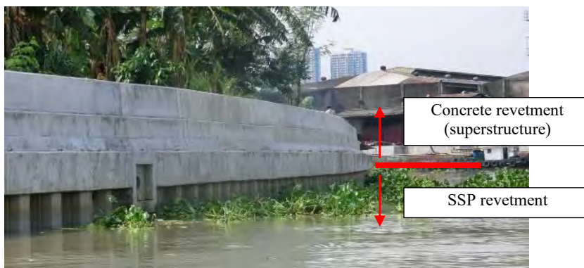
Figure 6.1.16 Example of Standard Revetment Structure Applied in Sta. 6+700 to Sta. 10+500
