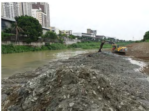
Figure 5.2.18 (Photo) Riverbed excavation
