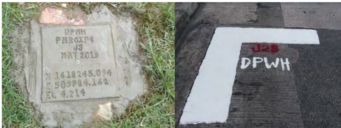
Figure 5.1.3 Examples of Control Points Established in this Detailed Design
