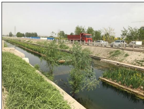
Irrigation Channel near a Sewerage Treatment
