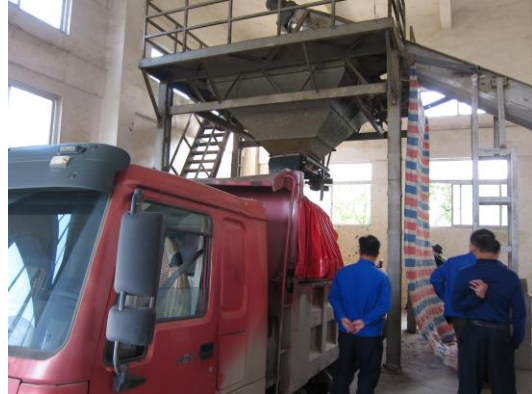
Truck for taking out sludge
