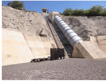
(1) Penstock pipe and (2) the power station
