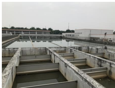
Chengbai Water Treatment Plant
