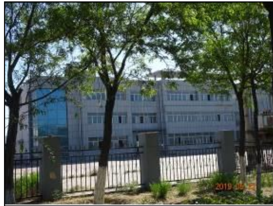
Plant Left Unattended in an Industrial Development District (Shizuishan City)
