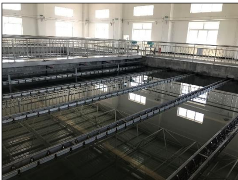
Huinong Purification Plant Prepared built under This Project
