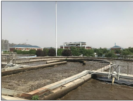
5th Sewerage Plant Constructed under This Project
