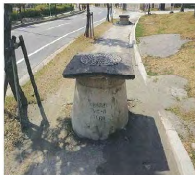
Fig. 6-78: Manhole floating due to soil liquefaction during the Great East Japan Earthquake (March 11, 2011 in Urayasu City, Chiba Prefecture) (Source: Miwa Horii)
