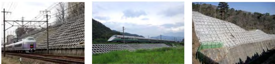
Fig. 6-21: Cribwork by concrete spraying to prevent landslide (Left: Chuo main line, Center: Yamagata Shinkansen, Right: Cribwork for natural slope (Source: JR East)
