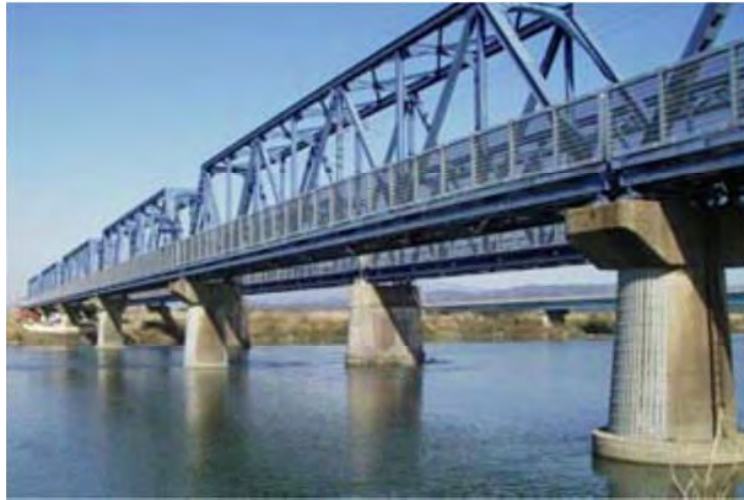
Fig. 6-22: Installation of perforated metal fences for wind power reduction: (Uetsu Main Line, between Sagoshi and Kita-amarume (Source: JR East))
