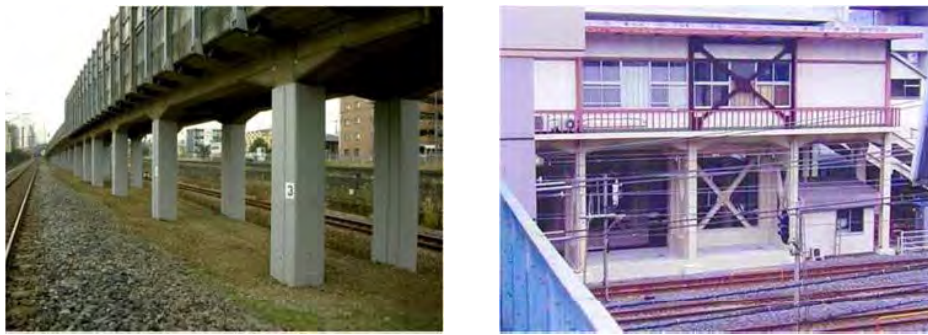
Fig. 6-19: Reinforcement of viaducts and station building (Source: JR East)
