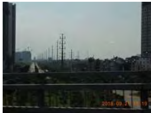
Mono-pole transmission line observed from tw-1 toward Chem SS
