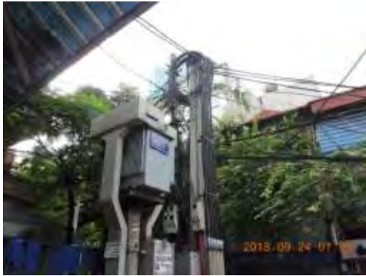
Distribution transformer on elevated concrete foundation
