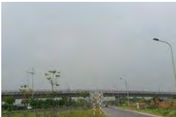
Location crossing Nguyen Khe Flyover
