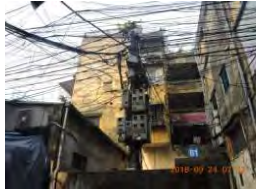
Congested LV distribution lines and power meters
