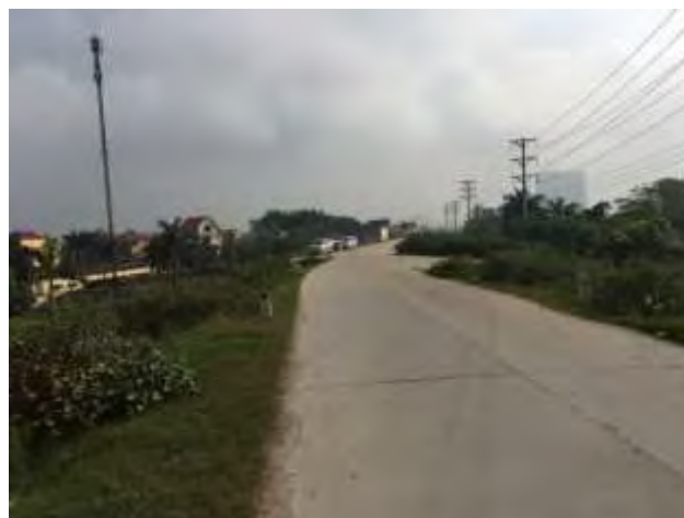
Figure 16-13. Present Conditions of type the Red River Left Dyke Road
