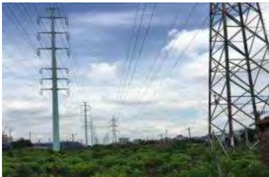
Location crossing 110kV line (Ciputra)
