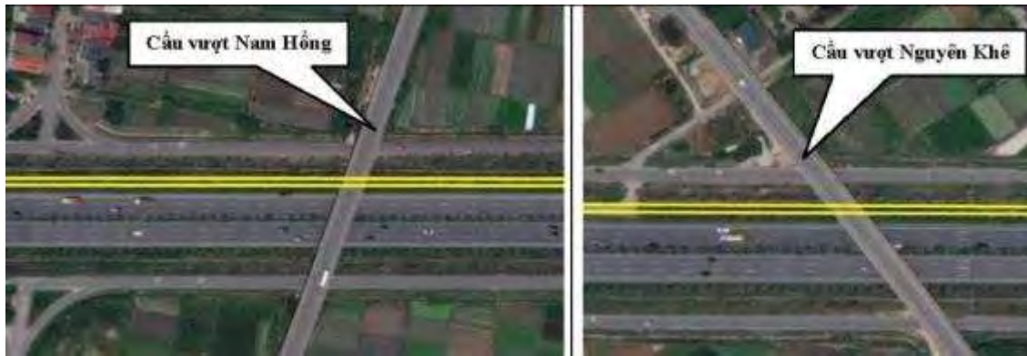
Figure 6-9. Intersection with Nam Hong and Nguyen Khe Flyovers
