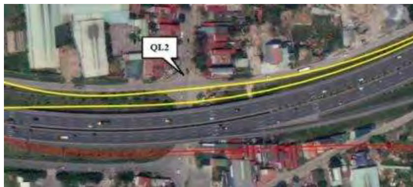
Figure 6-11. Intersection with NH2
