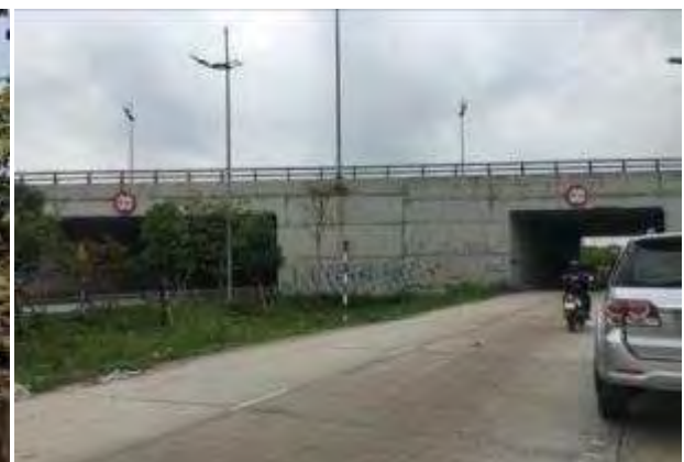
Location crossing over NH-18
