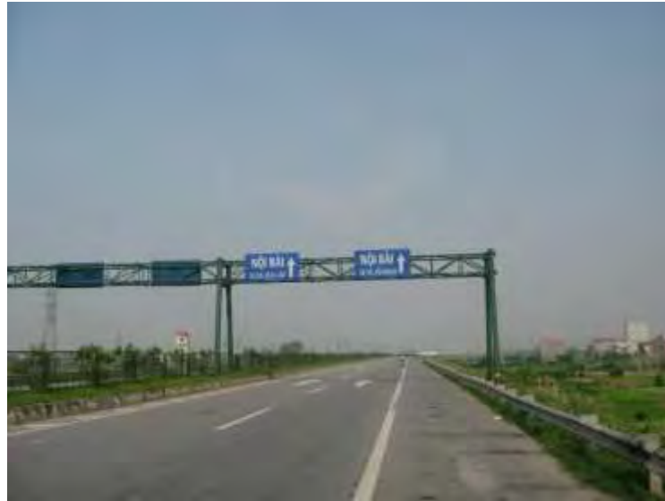
Figure 16-9. Present Conditions of National Highway 18
