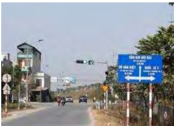
Location crossing over NH-2
