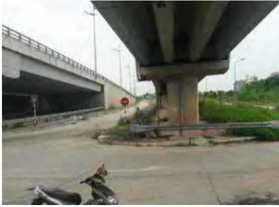
Location crossing Ring Road 3
