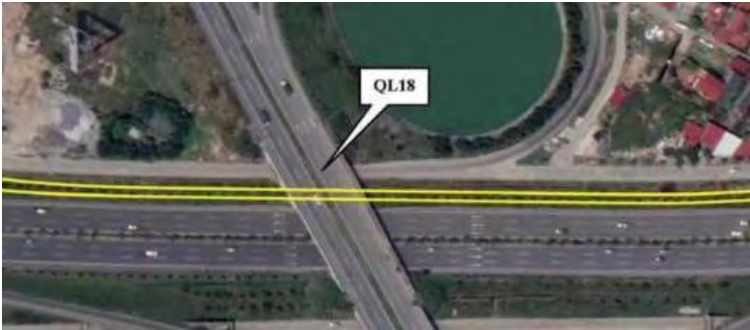
Figure 6-12. Intersection with NH18
