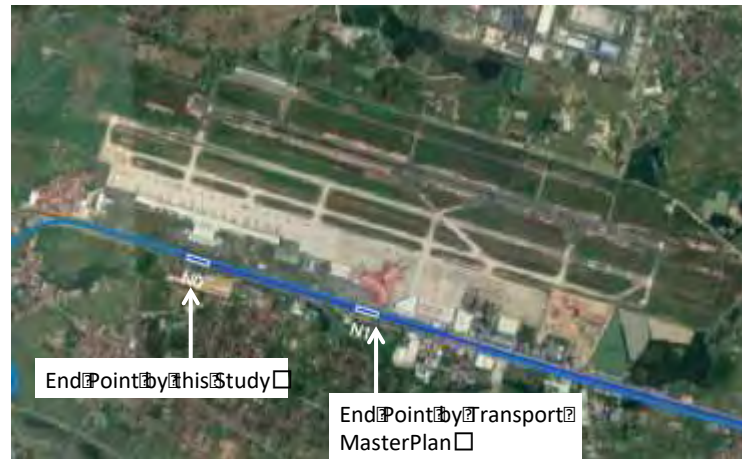
Figure 6-7. Ending Point of Line 2.3
