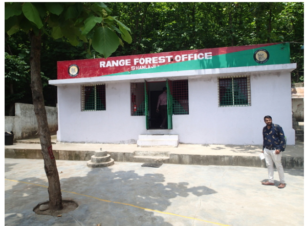
Exterior appearance of Shyamlaji Range Office in Aravalli Division
