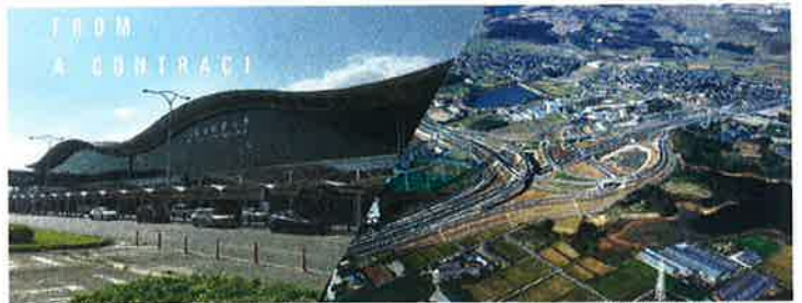
Saitama International Airport
