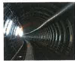
Taipei's Subway Network Songshan Line (Taipei City, Republic of China) Construction of three stations and six tunnels located in the financial district of the downtown area in the largest concrete structure of the Taipei Metro Songshan Line. It was many awards including Taipei City's award for excellent construction site management.
