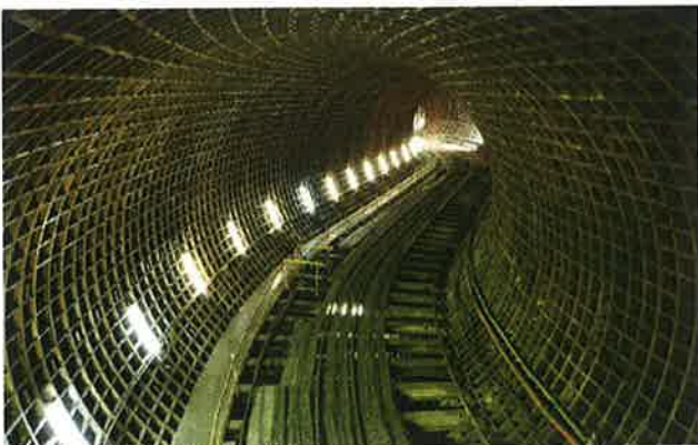
Katsushika Pump Station (Katsushika Ward, Tokyo) Construction and upgrade of pumps in Tokyo's Katsushika pump station. Its objectives are to prevent inundation of the Tachikawa River basin and improve the water quality of the Katsushika Canal. Length of total station, 80 m length, and 1,500 m 2 finished inner diameter.
