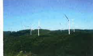
Suzu Wind Power Plant (Suzu City, Ishikawa Pref.) Manda was involved in an EPC (engineering, procurement, and construction) contract in the development process for 26 wind power generators ranging from research and design to performance, transportation, and mounting and electrical work. They each have a total height of 100 m, a rotor diameter of 70 m, and a rated output of 1,500 kW.
