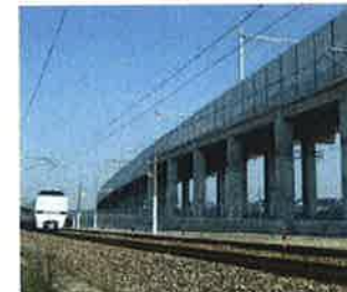
Hakuba Shinshansen Line (Hakuba Station, Nagano Pref.) Construction of the viaduct between the points at distances of 300,000 km and 200,000 km from the Hakuba Shinshansen Line, Imabishino, NC. It included concrete rigid-frame viaduct, NC abutments, NC bridge piers, RC girder, RC girder, and concrete girder, and subgrade work.
