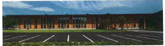
Susaia Town Office (Susaia Town, Kanon District, Iwate Pref.) (West 5th BCS Prize) Parks and green areas are being constructed by using L&L and local materials and locally manufactured and processed timber. It has advanced design from shared work between local housing bodies while maintaining a traditional layer of pure wooden architecture.
