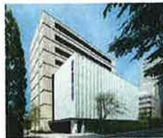
Osamu Gakko Educational Institute Osamu Women's University Building II (Chiyoda Ward, Tokyo) School building aimed at further expanding and enriching the educational environment of the Institute's Chiyoda campus, with an eye towards their "Education for Construction for people," "Education for the environment," and "Education for the future." It is an eight-story measurement building with lecture rooms, laboratories, computer rooms, study rooms with computers, student rooms, etc.
