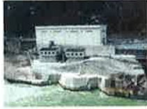
Toyomi Hydroelectric Power Plant (Miyagi Pref., Higashikantoku District, Miyagi Pref.) The hydroelectric power plant, constructed in the left bank of the Arima River from 1977 to 1979, was substantially expanded to increase its maximum output from 56,400 kW to 11,700 kW by upgrading the efficiency of equipment while adding existing facilities such as the dam and fish passages.
