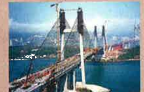
Kap Shui Mun Bridge Completed in 1981, the 1,000-meter-long bridge and the Kap Shui Mun Bridge in Hong Kong, both of which were completed by Maeda, are said to be the longest and the highest bridge in the world.
