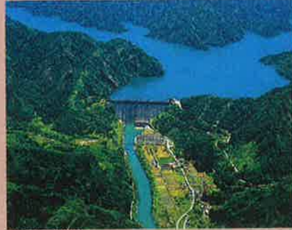
Tagokura Dam (Philippines) Completed in 1986, the dam height and length are 145 meters and 492 meters, respectively, with gross average capacity of 416 million cubic meters. It is the largest dam in the Philippines. It is the largest dam in the Philippines.
