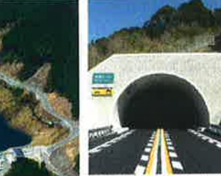
Higashi-Kyushu Expressway (Shiki Tunnel) (Fukuoka City, Fukuoka Pref.) Manda tunnel constructed by mixing excavation with a length of 300 m. People in the tunnel area of East Kyushu were looking for an early opening because of their need to improve traffic in major cities in Kyushu. It was opened in March 19, 2014.
