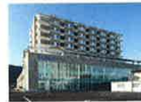
Teikyo Hospital (Fukuoka City, Fukuoka Pref.) Construction of hospital facilities that serve as Teikyo Hospital's medical infrastructure. The hospital has a specially designed system for infection control and also has a meeting hall. It is a nine-story building with a total floor area of about 30,270 m 2 and 600 hospital beds.
