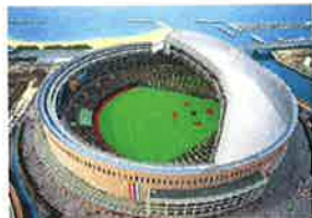
Fukuoka Dome (currently, Fukuoka Yafexhal Dome) (Fukuoka City, Fukuoka Pref.) First and only baseball game in Japan which has a retractable roof. The 12,000-ton heavy roof consists of three panels and fully opens or closes in approximately 30 minutes by rotating both of them right and left by 120 degrees.
