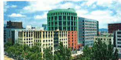
Hyatt Regency Fukuoka (Fukuoka City, Fukuoka Pref.) Hotel Regency Fukuoka, formerly designed by well-known architect Perini, and with various facilities including office buildings. It received the 26th BCS Prize.
