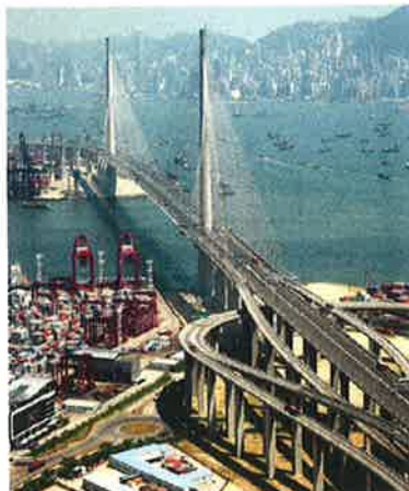
Zhongshan Bridge (Dong Kong) One of the world's largest cable-stayed bridges, which links Shau Kei Wan Island and Tsim Sha Tsui Island. The length of its main span, main span, and total length are 261 m x 2, 1,118 m and 1,390 m, respectively, and it has two main bridge piers (270 m high above sea level).
