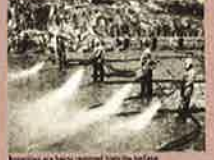
Excavation is being carried out on the dam.
