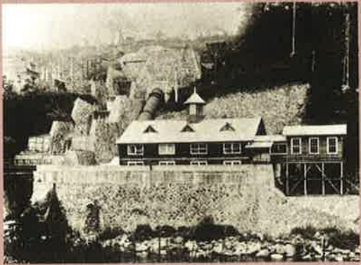
As a construction site of the Kiso Fukuishima No. 2 Hydroelectric Power Plant, Maeda Maeda Co., was in the center of the scene.
