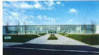
Akasaka Crystal Wing (Minami City, Saitama Pref.) (West 4th BCS Prize) Architectural design by the headquarters office in its Minami place. It has a large common space of approximately 2,000 m 2 created by using 11 strong beams with a length of 22m.
