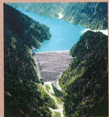
Takase Dam (Japan) Completed in 1978, the dam height and length are 176 meters and 303 meters, respectively, with gross storage capacity of 16.1 million cubic meters. It is the largest dam both under the Takase River Redevelopment Project.
