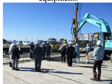
Picture 19. Train the construction management method
