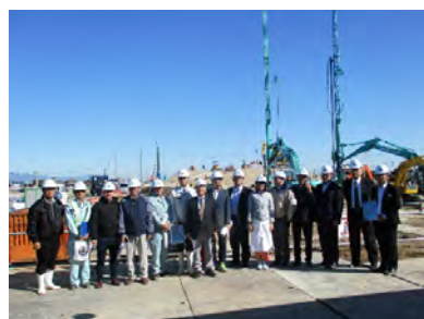
Picture 18. Inspect the construction site of MITS method
