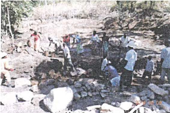
Construction Site of Kapanda Permanent Weir (Kasama District, Northern Province)
