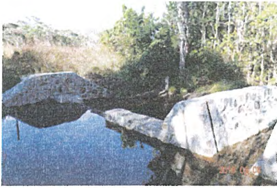
Mpela Permanent Weir (Mporokoso District, Northern Province)
