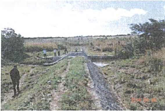
Musanza Permanent Weir (Nakonde District, Muchinga Province)
