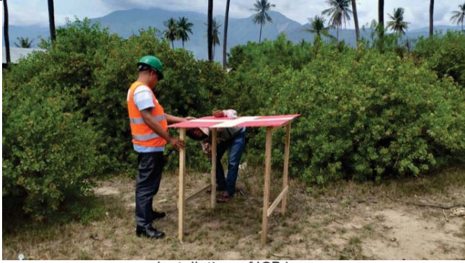
Installation of ICP box
