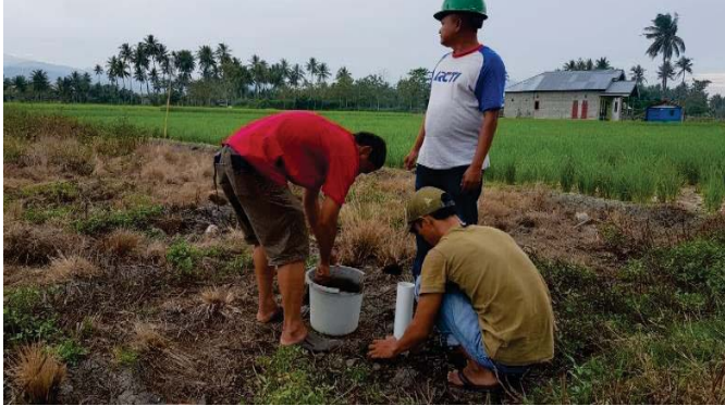
Base Point installation
