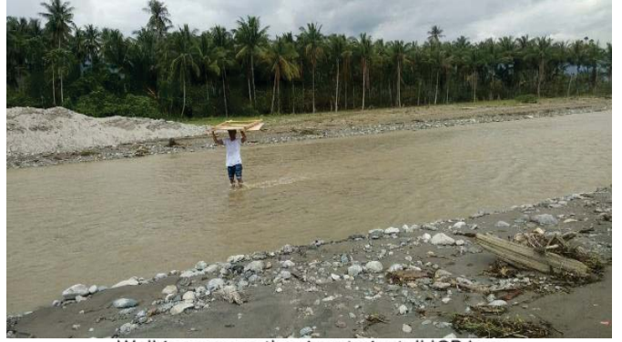
Walking across the river to install ICP box
