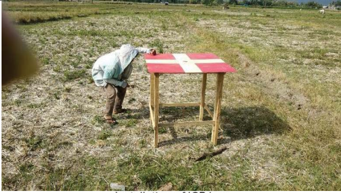
Installation of ICP box
