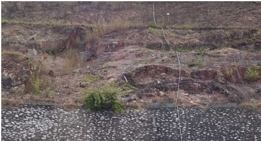
Before Construction (2018-Sep.)
