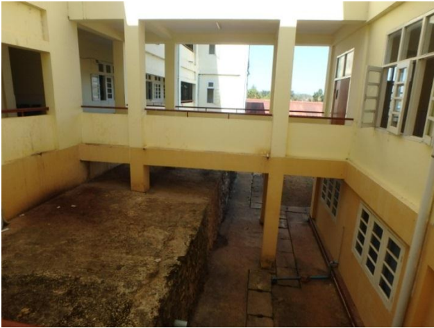
Connecting corridor between Building A1 and A2 (Constructed in 2004)
