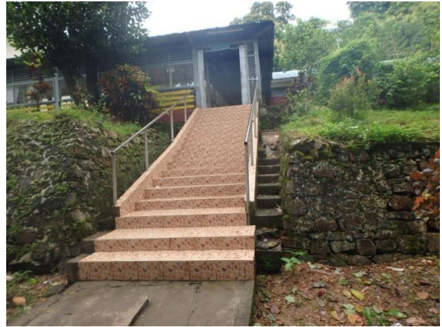
Stairs connecting to Medical ward (Constructed in 1994)
