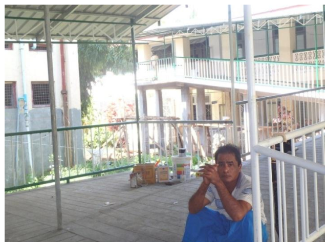
Slope in the new building under the construction (Gradient on the slope is approximately 1/10)
