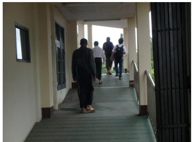
Steep slope connecting between ICU and Operation theatre
