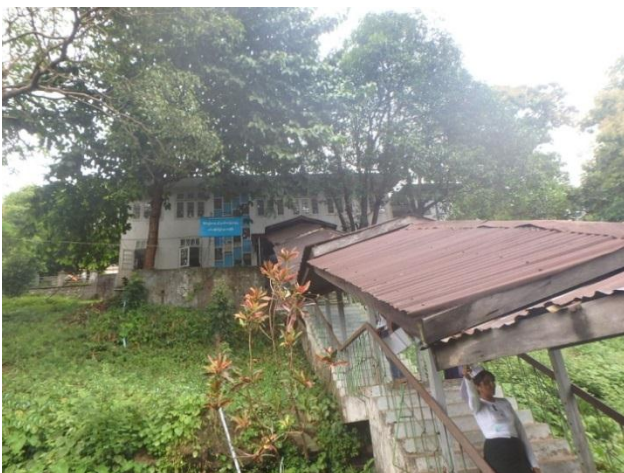
Stairs connecting between Psychiatric ward (Constructed in 1982) and Medical ward (Constructed in 1994)
