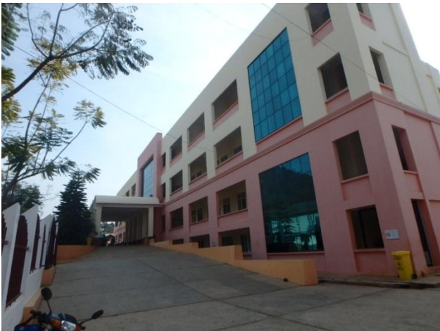
Building no.3 for OPD, Operation theatre and Delivery room (Constructed in 2007)
