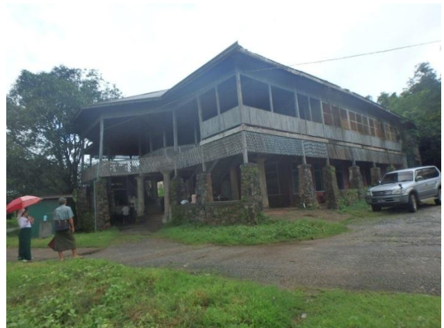
MOUNT HOPE constructed a hundred years ago. Wooden parts of first floor have been getting rot and currently not used.
