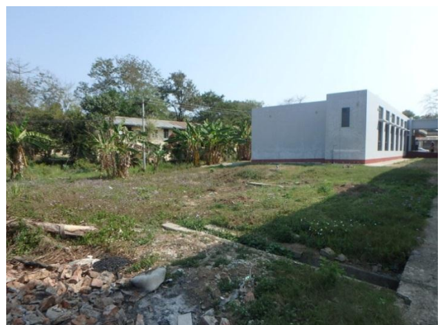
Building for CT scan room constructed by Japanese aid (Constructed in 2014) and Wadi passing in the hospital
