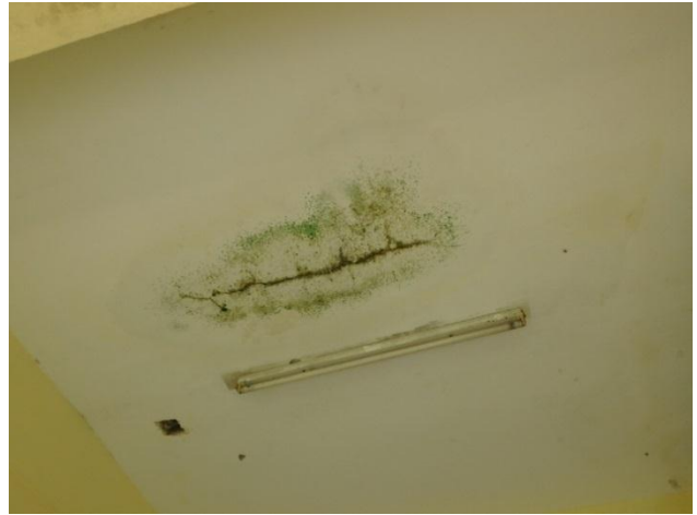
Corrosion of reinforcing bars of floor (Constructed in 2003)
