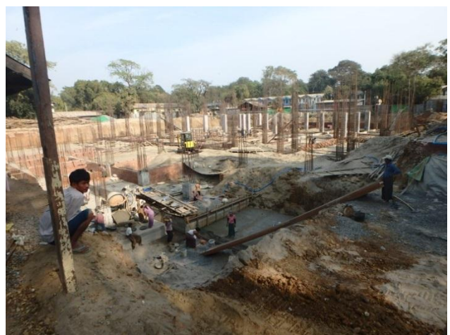
New 6 stories building under construction for OPD and Operation theatre
