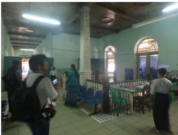
Wooden parts have been getting rot at Ob and Gyn ward (Constructed in 1917)
