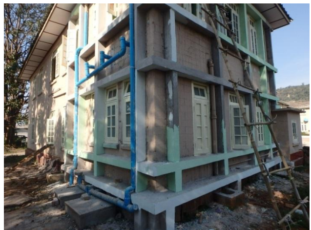
Renovation work for Pediatrics ward (Constructed about 100 years ago)
