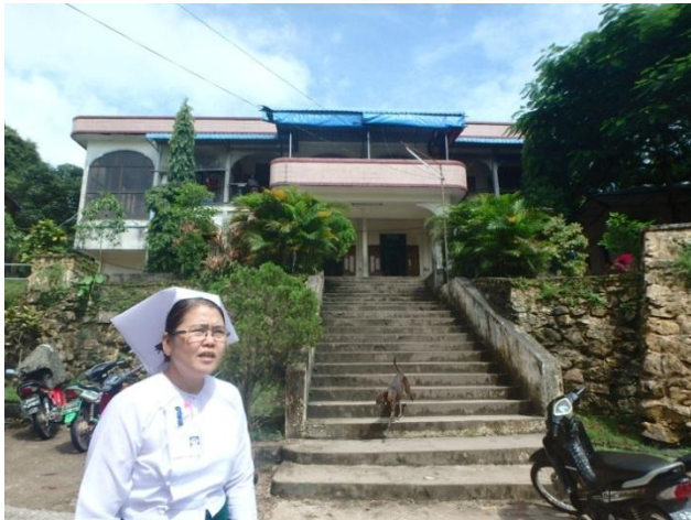
Stairs connecting to Pediatrics ward (Constructed in 1965)
