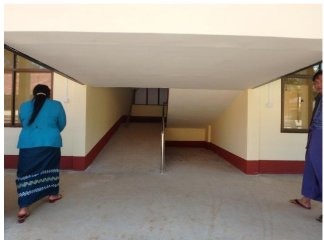
Steep slope in the new building for OPD and Medical ward (Gradient on the slope is approximately 1/7 to 1/8.)
