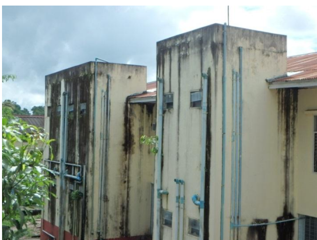
Toilet's roof with water tank and sloped roof of Building D
