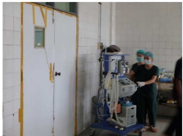
Doors of Operation theatre sealed with plastic tape (Lack of airtightness of room)
