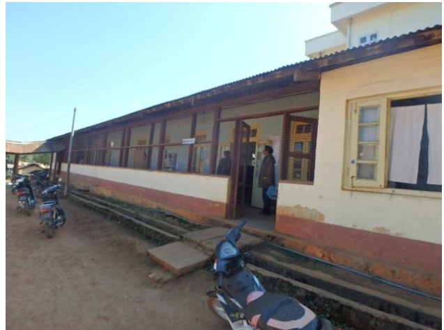
Building for Medical care ward planned to be demolished (Constructed in 1946)
