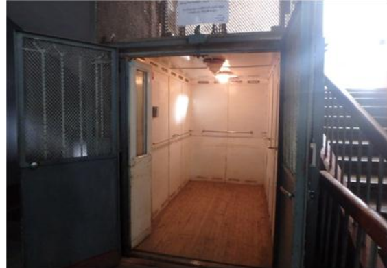
Elevator constructed in 1961 and still properly working in the main building
