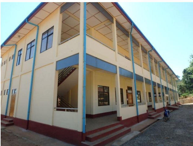
New building for OPD (Ground floor) and Medical ward (1 st floor) (Constructed in 2014)
