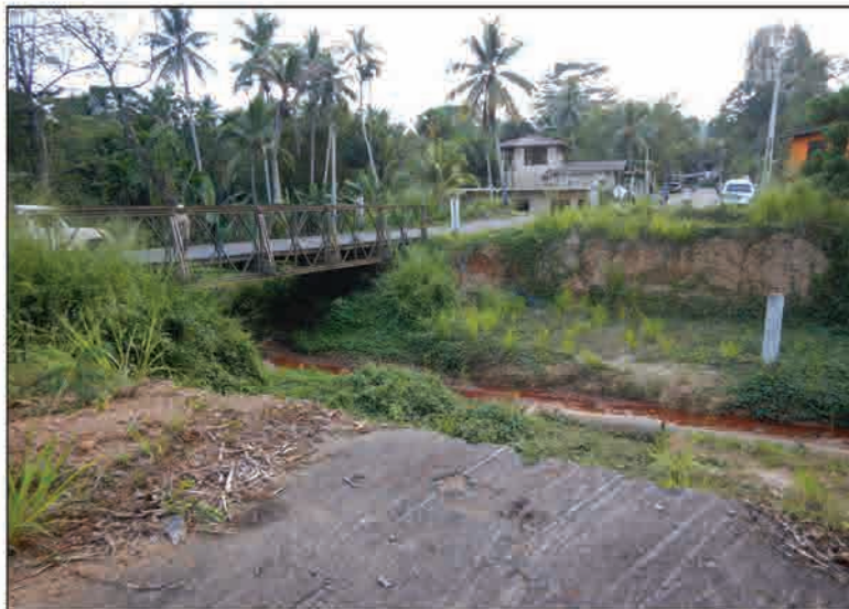
P2 The temporary bridge built before the debris flow occurring in 2017
