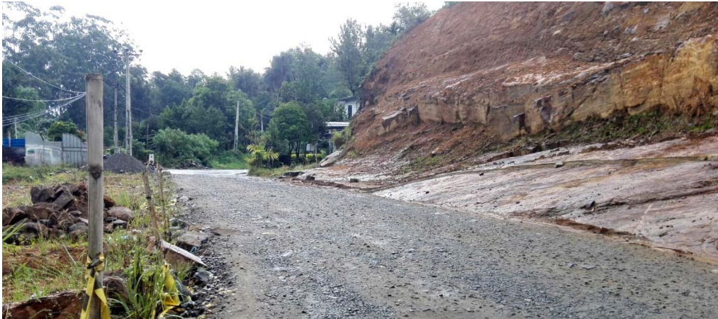
Site No.36: Route B149 9.0km-9.1 km (Maskeliya Hatton Delhouse Road )
