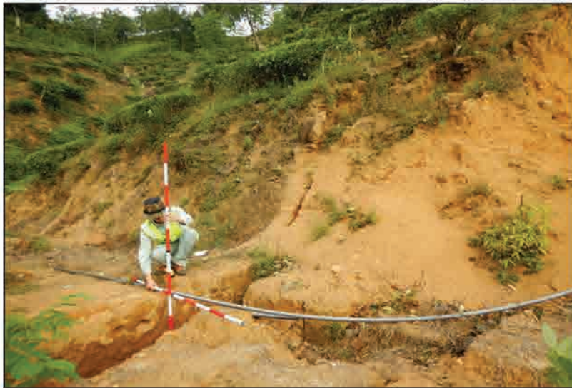
P2 The failure scarp and cracks along the slope failure
