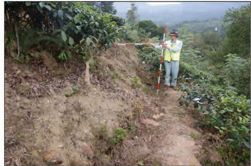
P4 Stepped landform above the slope failure, showing potential instability toward the upper slope
