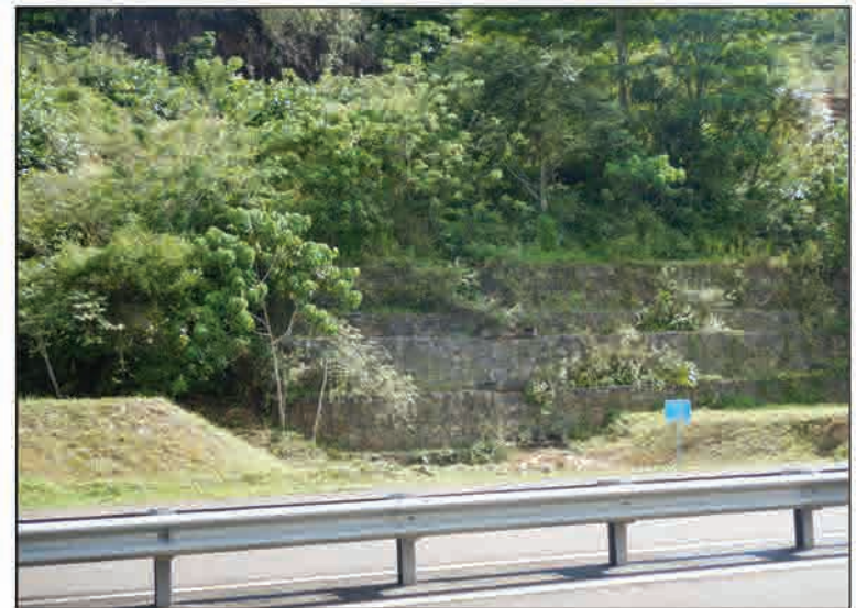
P3 The installed gabion retaining wall near the slope failure
