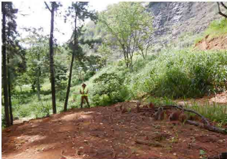
P3 The lower slope the landslide below the road
