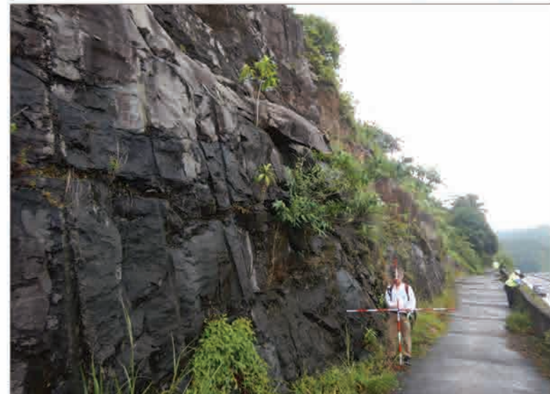
P3 A village road at the middle of rock cut slope, showing well-developed dip slope
