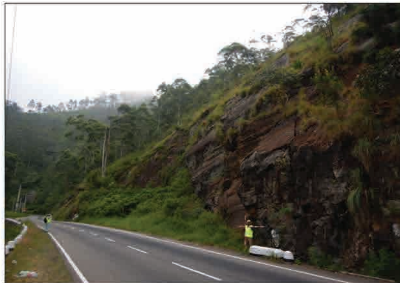
P6: The cut slope of bedrock
