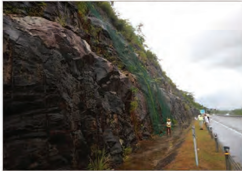
P5 Highly fractured rock mass and emergency nets installed by RAD
