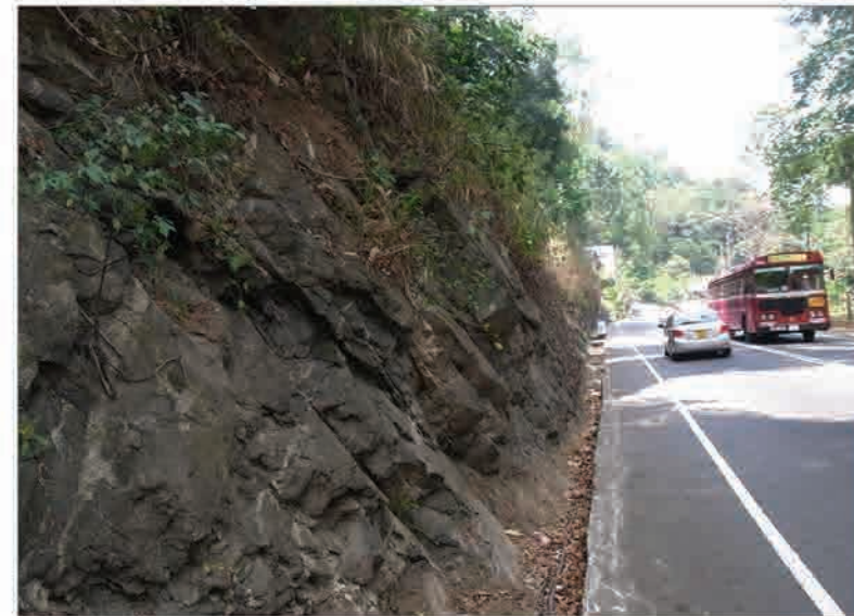
P4 Foliation joints dipping adversely out of the slope.
