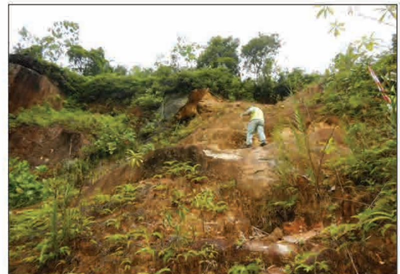
P4 Main scarp of the slope failure, showing the strongly weathered rocks
