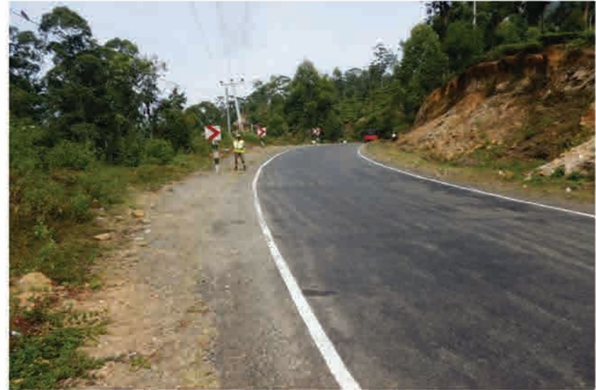
P2 The upper slope of the landslide area looking from the ending point of the road
