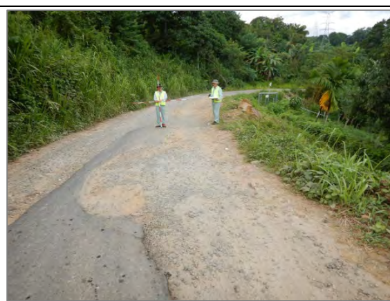
Photo 10: Field survey for preliminary design (Land slide site).
