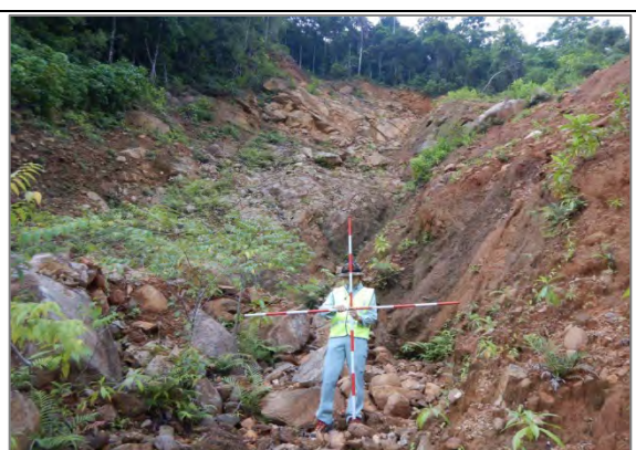
Photo 11: Field survey for preliminary design (Slope failure site).
