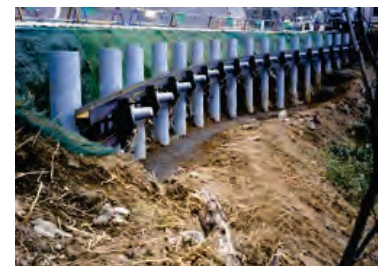
Steel pile with ground anchor (Source: Isabou.net)
