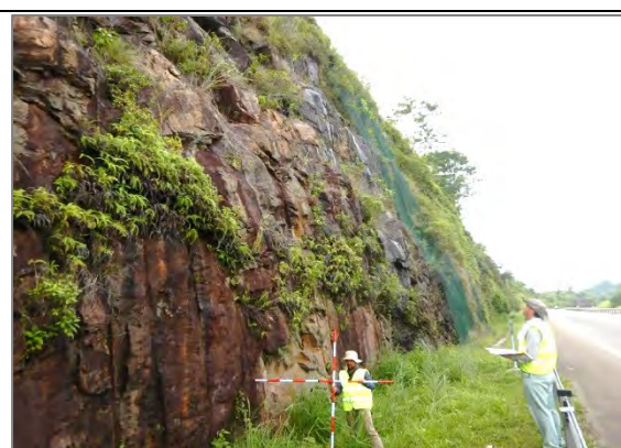
Photo 12: Field survey for preliminary design (Rock fall site).
