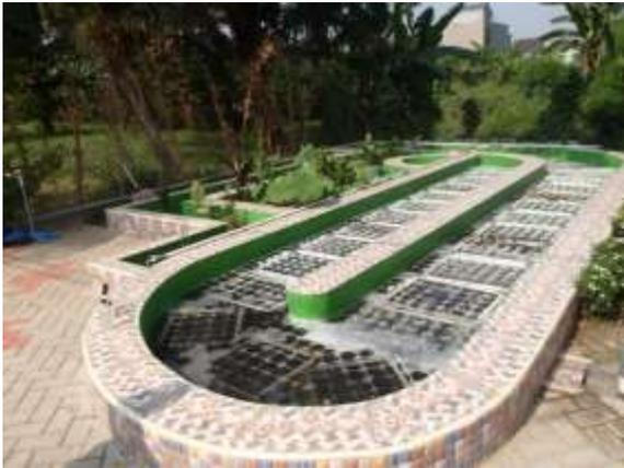
**Fig. 3-35 Biocord treatment system with aeration**
