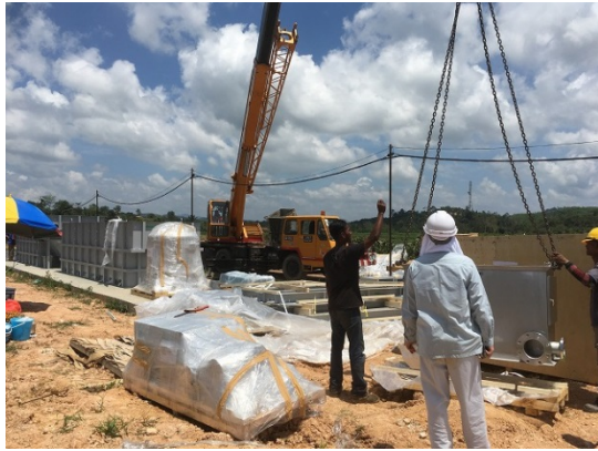
Installation Work (March 2018)
