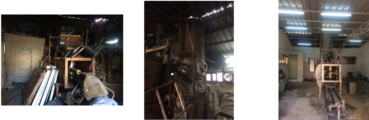
Figure II-10: Rehabilitation of Al Shifa Hospital Incinerator in Gaza (Before and After)
