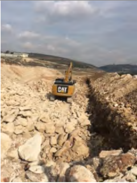
Construction works in new leachate pond (2018)
