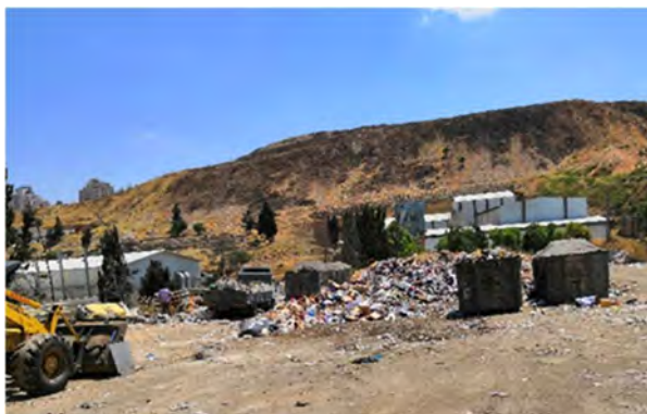
Ramallah Waste Transfer Station
