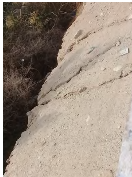
Photo (8)- Cracks in the retaining wall
