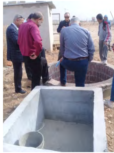
Photo (6) – construction of pilot Anaerobic Digestion system
