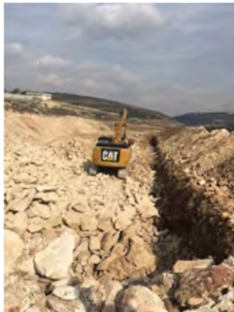
Excavation works for construction of new leachate collection pond at Zahrat Alfinjan
