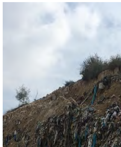
waste overturning behind the retaining wall-2018
