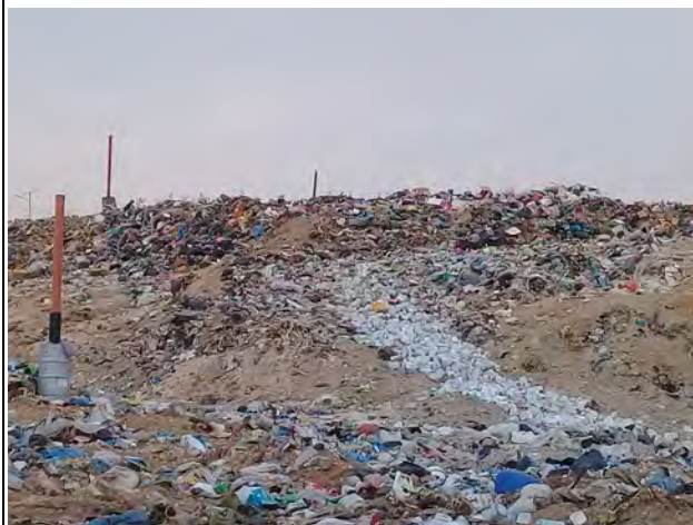
Soil Cover not Well Performed
