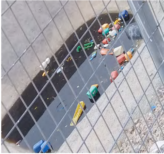
Photo (5)- waste accumulated in the leachate collection pond
