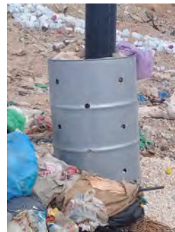
Photo (4) - gas ventilation
