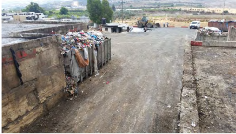
Waste Receiving Area in the Transfer Station
