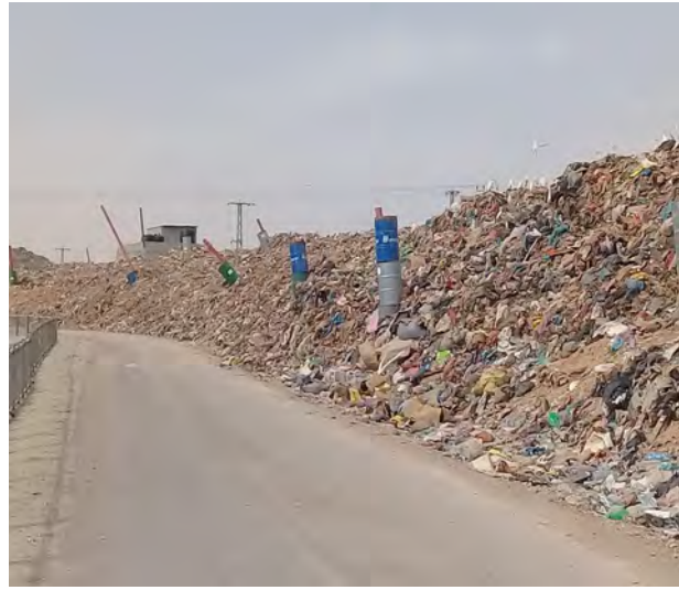
Gas Collection System in the new and old cells
