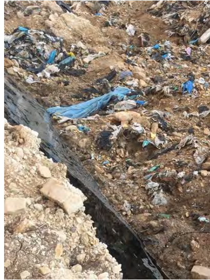
Leachate Overflow to outside -2018
