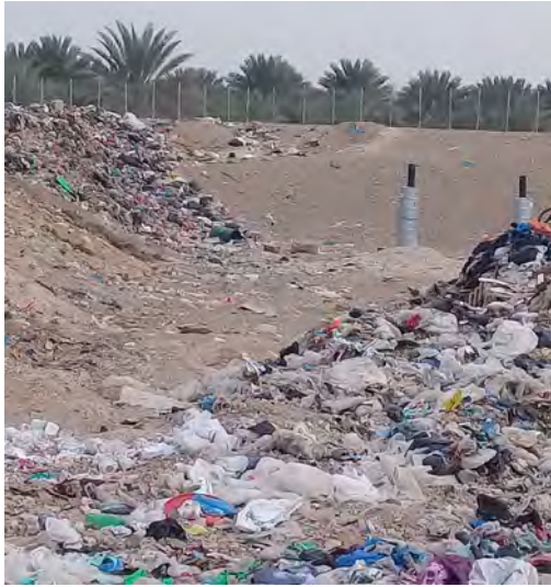
Gas Collection System in the new and old cells
