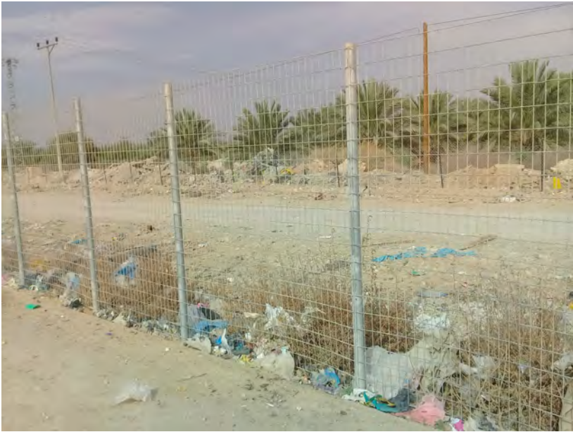
Waste Scattered around the Landfill site
