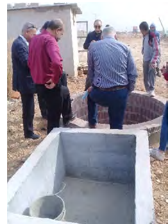
Construction of Pilot Anaerobic Digestion System at Jericho Landfill
