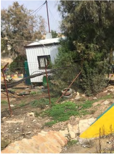
Storm Water Drainage ditch filled with -2018
