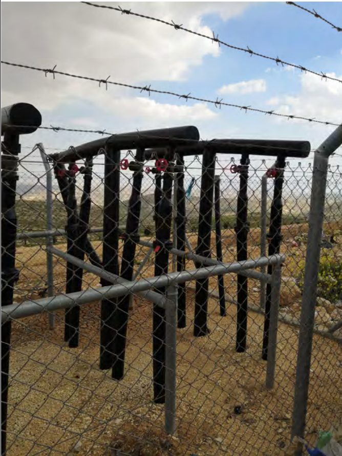
Gas Collection System in the new and old cells
