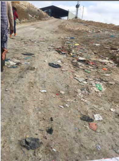
Internal road (Improperly paved and not clean)-2018
