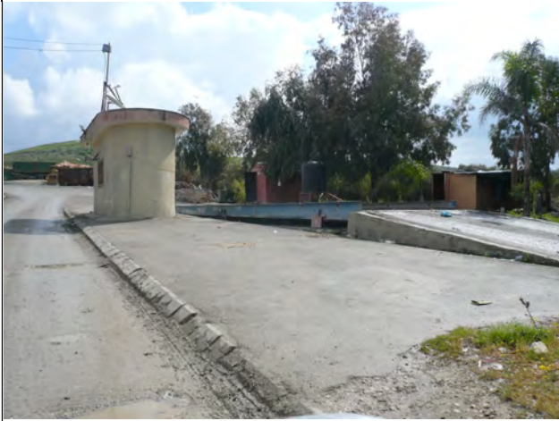
Weighing system and staff -2017
