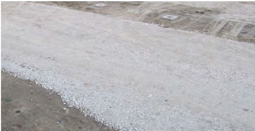
Figure 30: Under-construction street while filling with recycled aggregates
