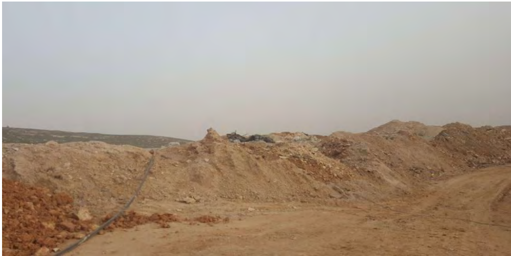
Figure 29: Piling of excavation materials to be reused in leveling a new road
