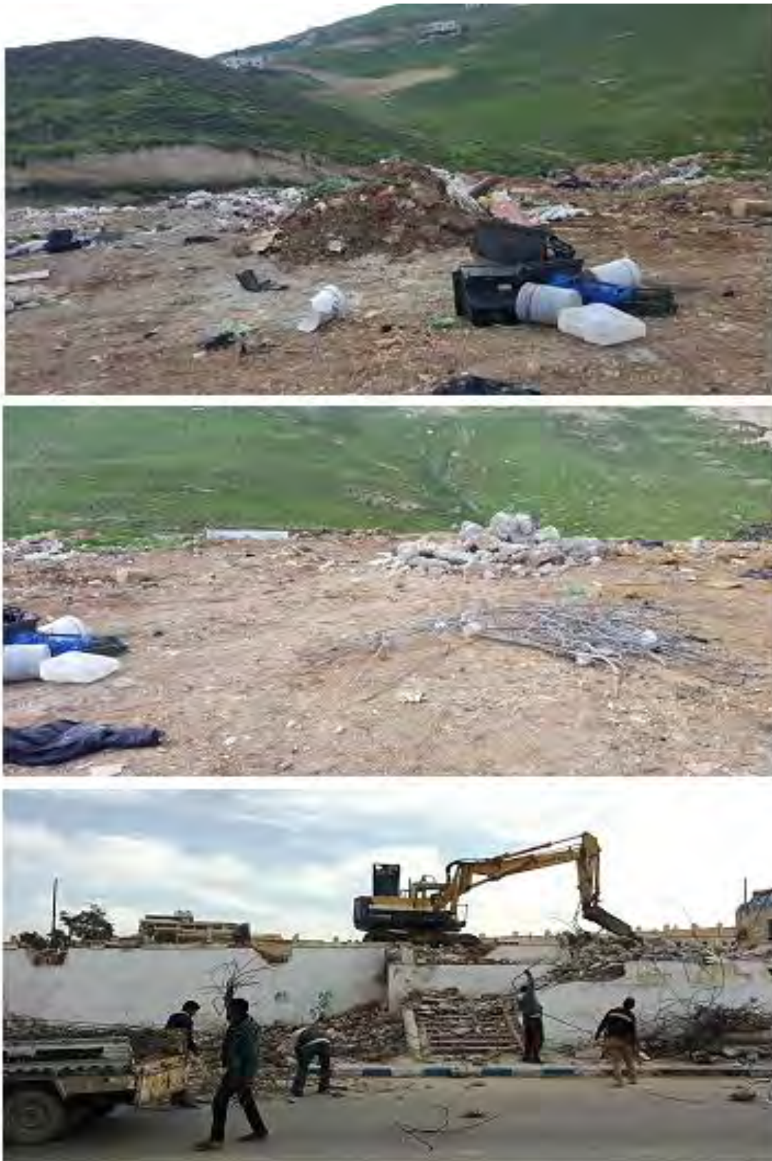
Figure 29: Separation of C&D waste components at different sites for recycling
