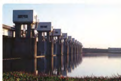
For River Water Level Control
