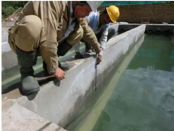
1-5 Leakage Test by Filling Water in Tank
