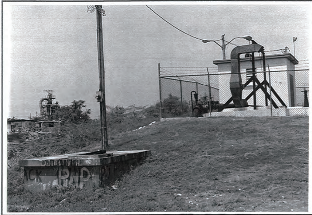
Plate 7 - New Haven pumping station.
