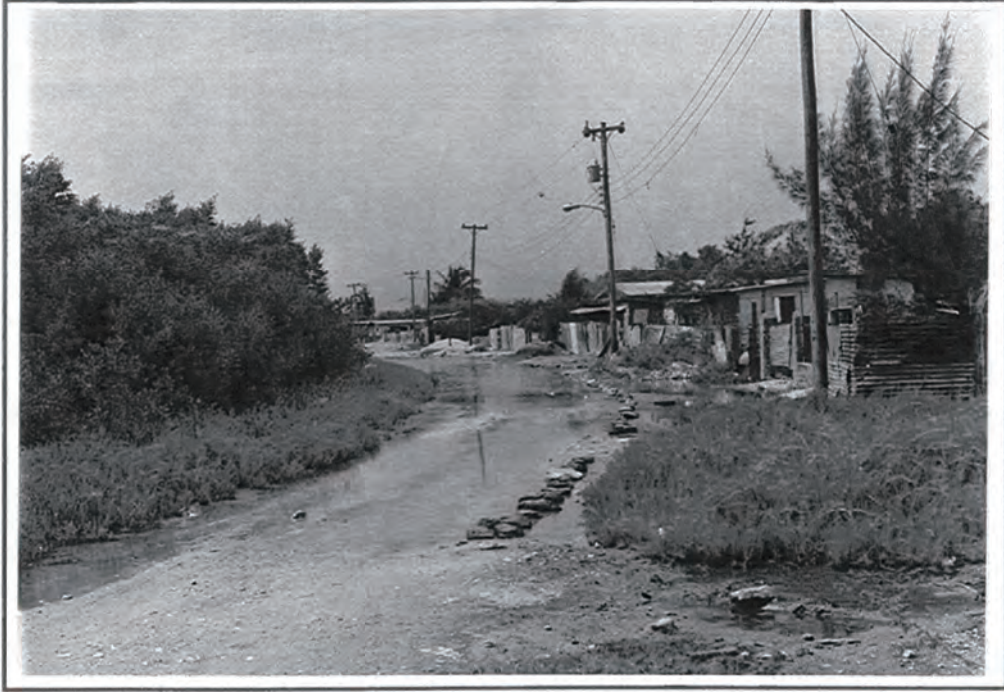
Plate 11 - The wetlands overflows onto the road in Riverside Gardens.
