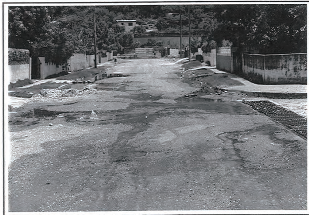
Plate 6 - Plates 4, 5, 6; Sewage emanating from surcharged sewer and entering storm drains. Note the retired Duhaney Treatment Plant in the background.
