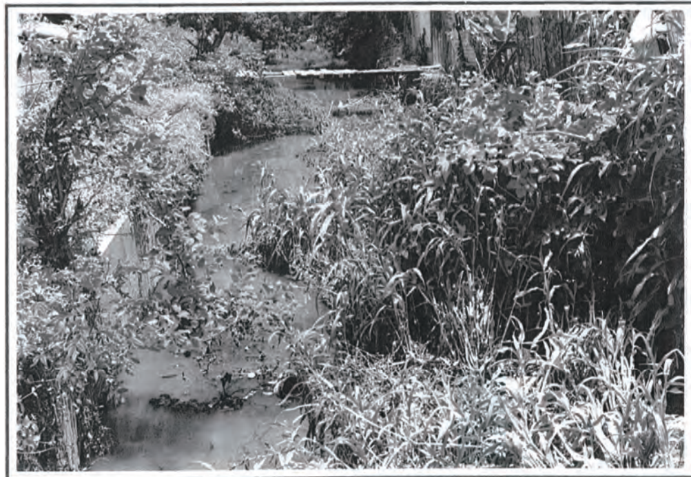
Plate 2 - Plates 1 and 2; The Northern Gully blocked with garbage and vegetation.
