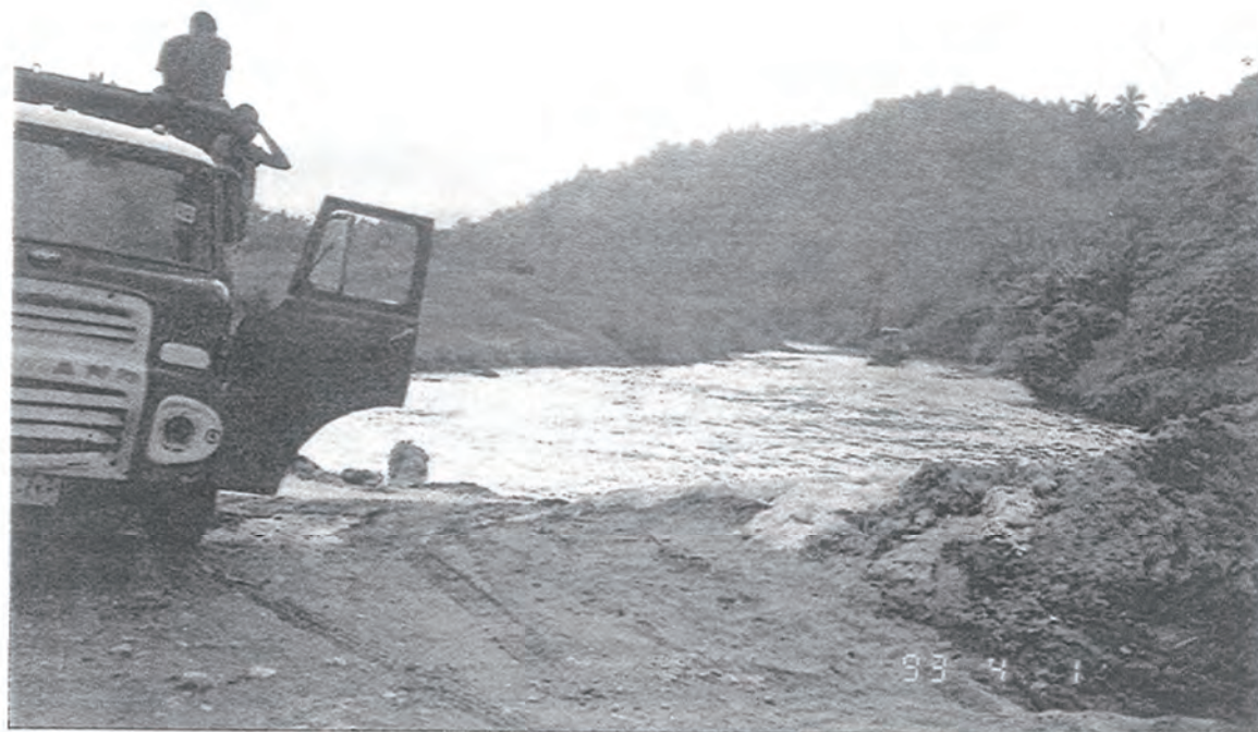
Plate 10 Sand dredging activities on the banks of the Rio Pedro.
