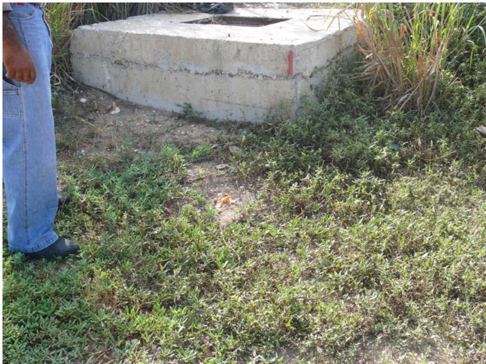
Photo 4 Close View of BM No. 1002
