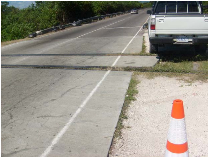
Plate 4 Picture showing existing site conditions. (Dyke Road)
