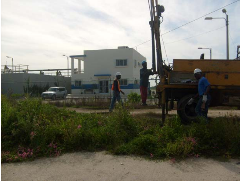
Plate 5 Picture showing drilling crew at work (Soapberry)
