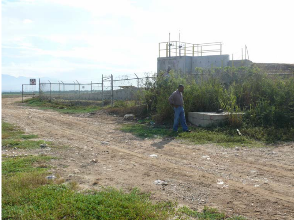
Photo 3 Distant View of BM No. 1002
