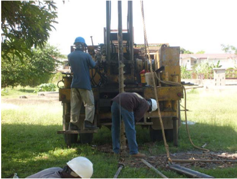
Plate 3 Picture showing drilling crew at work (Hamilton Gardens)
