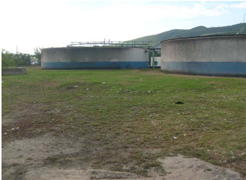
Plate 2 Picture showing existing site conditions (Bridgeport)
