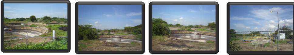
The General overview of the abandoned treatment plant facilities at the greenwich plant now pumping station
