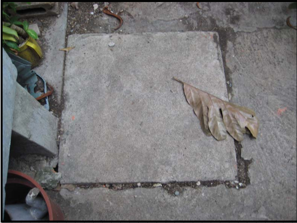
View of Closed Soak-Away Pit
