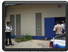
The general over view the facility at the Nanse Pen
