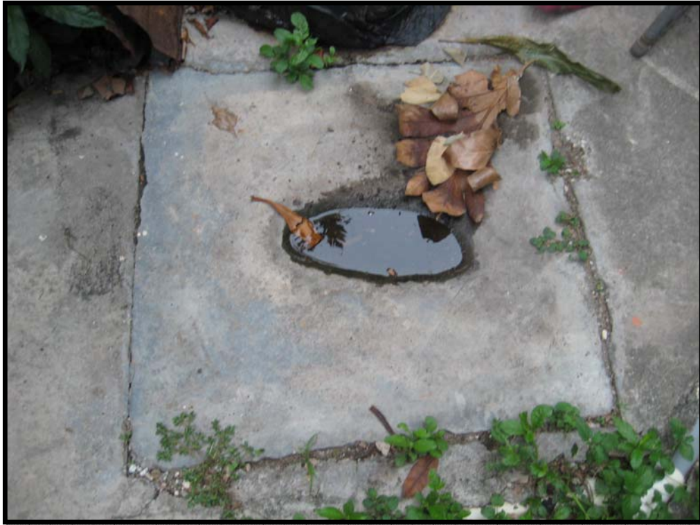
View of Closed Soak-Away Pit
