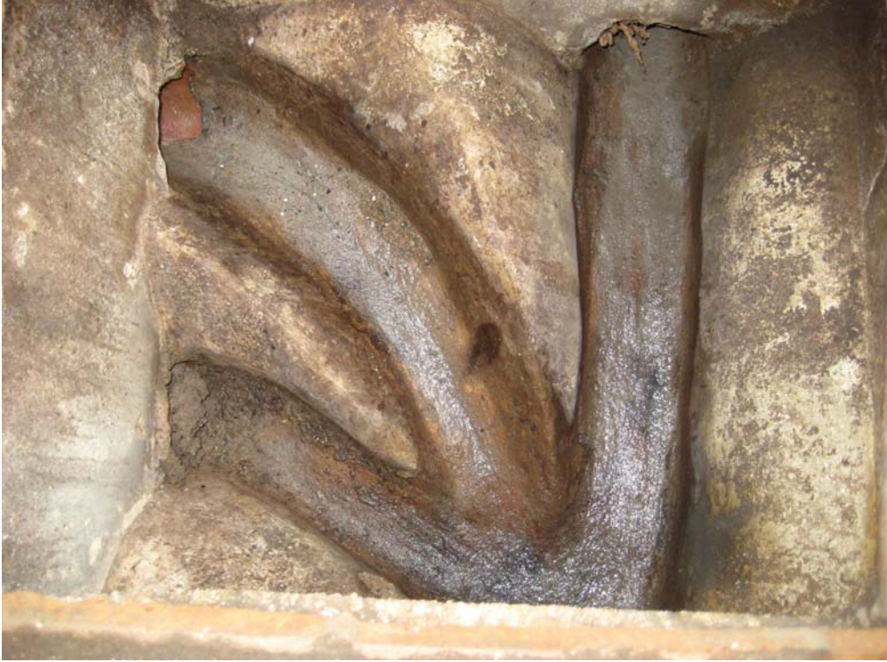
View of open Soak Away Pit
