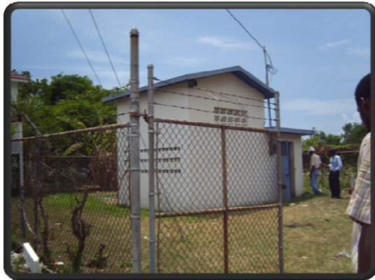
The above picture gives the general overview of the building which houses the pump units and the generator
