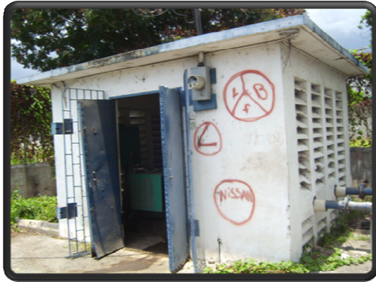
The above picture depicts the overall view of the much smaller Red Hills Rd. pumping station
