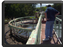
The above images depict the active contact tanks and the splitter box at the treatment plant
