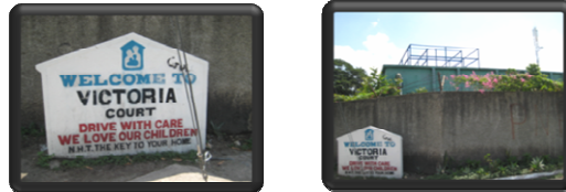
The above pictures depict the general over view of the facility at the Victoria Court's Treatment Plant
