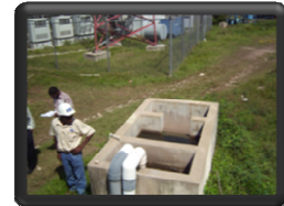
The above picture displays the inlet point and outlet point of the facility; Wet well, Clarifier, Automatic level Switch
