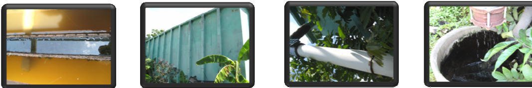
the above pictures depicts the outlet point and gives an idea of the TS level the leaves this facility
