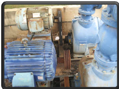
The motor that drives the Pump at the B.port Lift station
