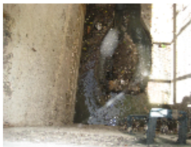
picture depicting the wet well and its screens which are currently blocked and is in need
