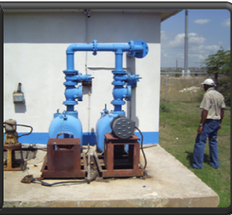
inlet pipe takes up waste from outside well directly below
