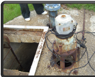
Access way to the wet well and vents at the Edgewater pump station
