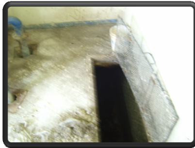
wet well at the facility covered with solidified grease
