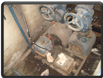
The motor which drives the pump unit
