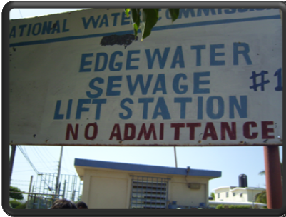
General over view of the facility at Edge water pumping station
