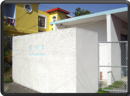
Building housing all the electrical, which should
