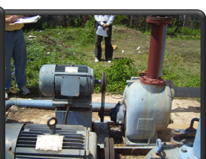
image showing the pipe to pump connection for the outlet pipes
