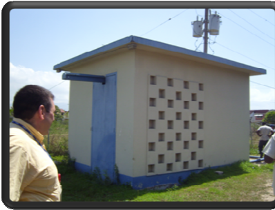
Building housing all the electrical, which should
