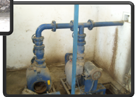
General piping layout at the Bridge View pumping station
