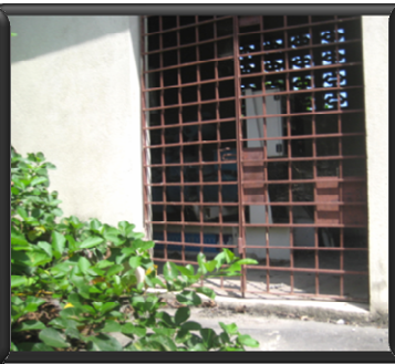
Building containing electricals and the
