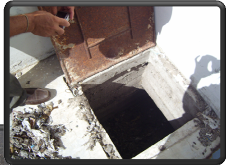
Outside cover to wet well of the Bridge View Pumping
