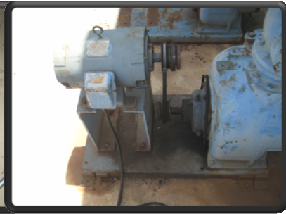
Motor for the back up generator inside the building
