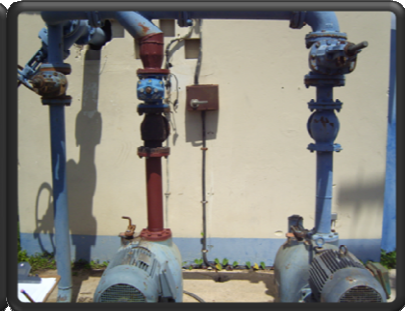
image showing the pipe to pump connection for the outlet pipes
