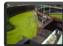
Pictures above displays the contact tank that is out of service at the Independence city plant
