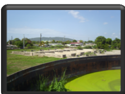
Pictures above displays the contact tank that is out of service at the Independence city plant
