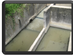
The above pictures displays the contact tank and the chlorination chamber
