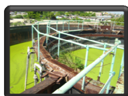
Pictures above displays the contact tank at the facility's northern end that is out of service at the Independence city plant
