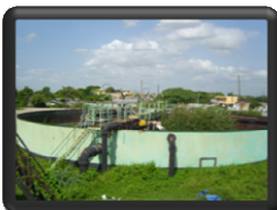
Pictures above displays the contact tank at the facility's northern end that is out of service at the Independence city plant
