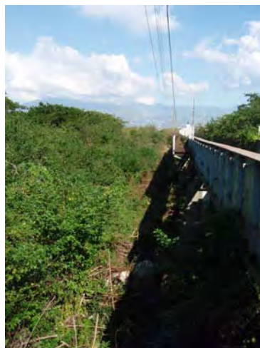
Figure 6.3.1 Site Condition for Pipe Bridge between Caymanas and Soapberry STP
