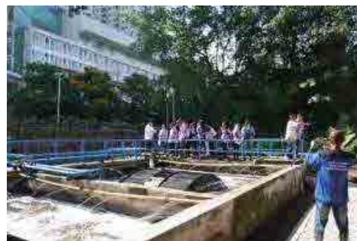
Sewage treatment facility at Waduk Melati
