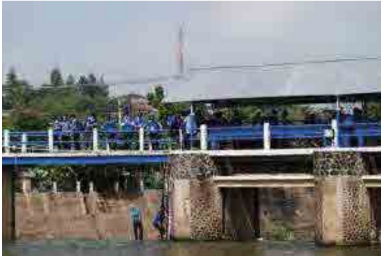
Field Study at Bendung Katulampa
