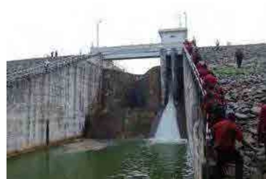
Dam body and Spillway of Situ Gintung
