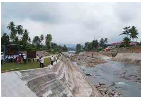
Photo-11 Sabo works at Batang Kuranji
