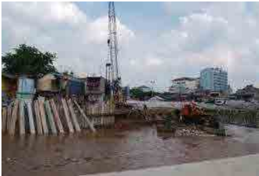
River Improvement works at Kampung Pulo
