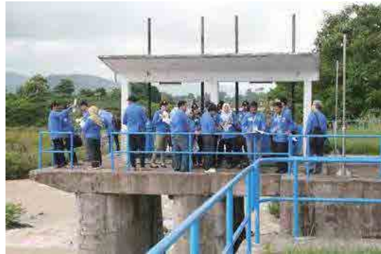
Intake Facility for Bili Bili Irrigation Area
