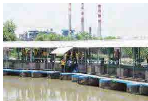
At Diversion Gates
