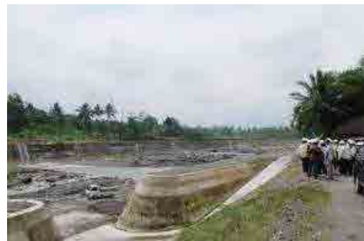
Photo-10 at diversion channel at Putih river
