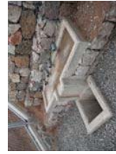
End portion of the drain pipe
