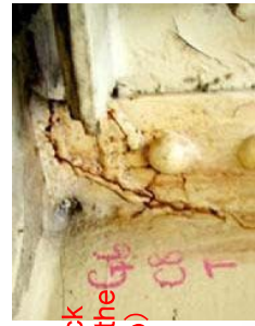
Fatigue crack (Advance to the back of web)
