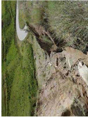
Damaged Road Shoulder
