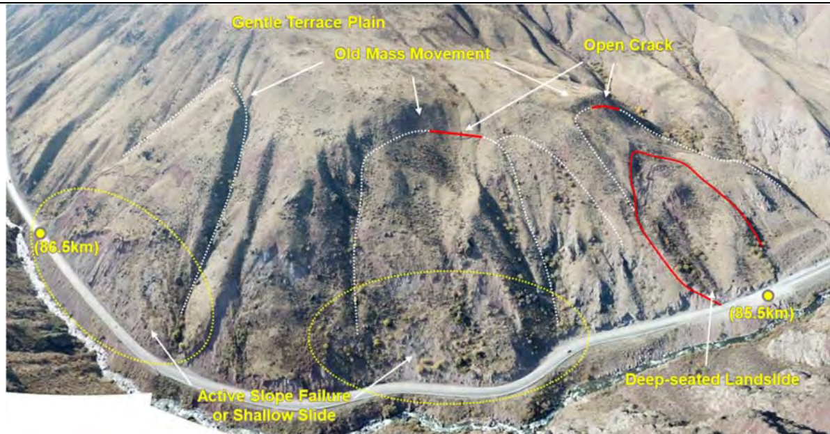
Figure 10-8 Outline of Drone Survey Target Area
