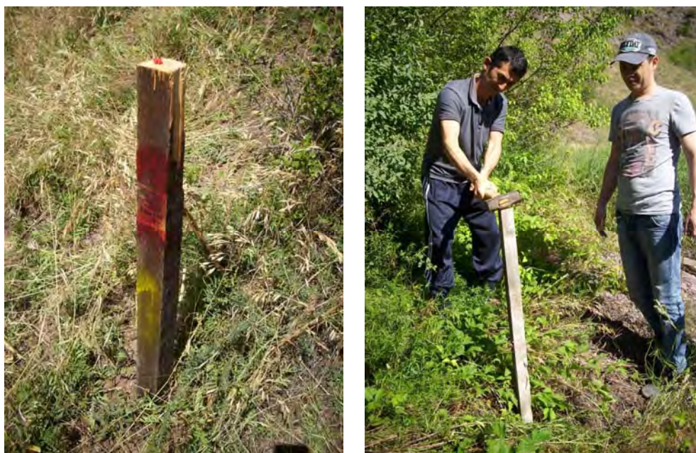
Figure 10-2 Install work of the wooden stakes (2016/6/29)
