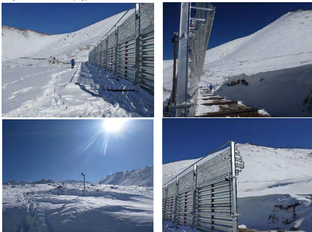
Picture 11-3 Installed Snow Fence as of October 2017
