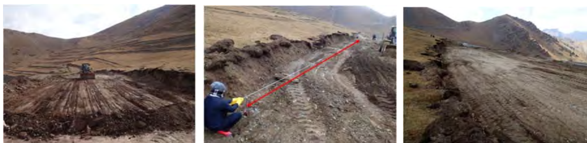
Picture 11-1 Construction Road
