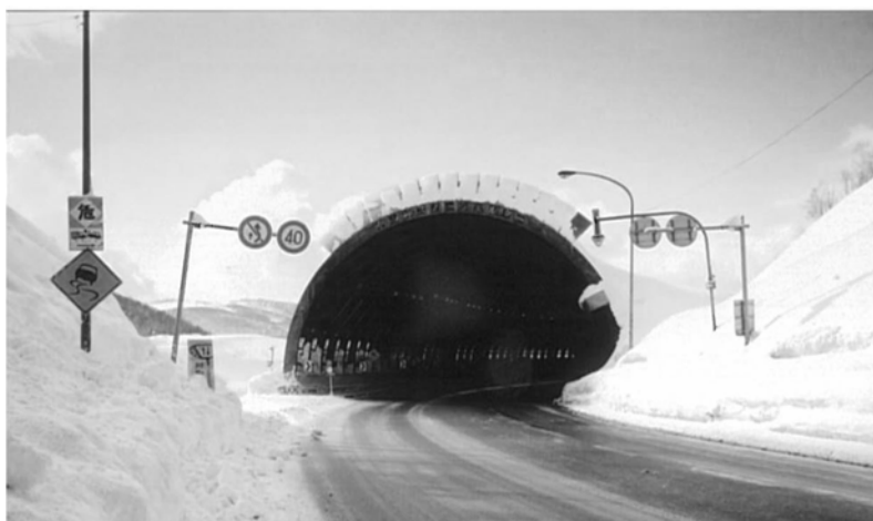
Picture 6-16 Snow Shelter
