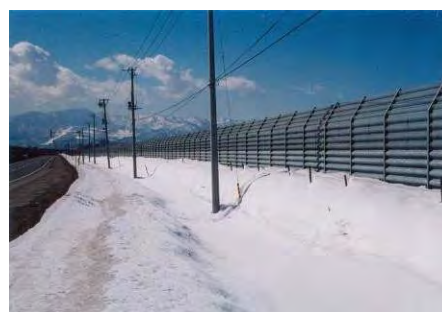
Collector Snow Fence
