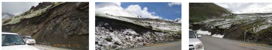
High Cut Slope
