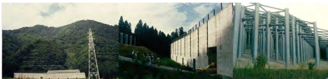
Protection Wall and Energy Dissipating Fence
