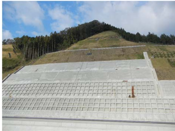
Figure 4.1-2 The view of slope protection measures along Japanese Highway
