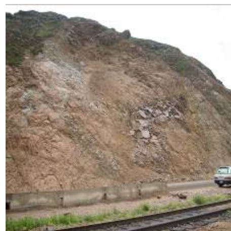
Slope Collapse from Road Shoulder to Lower (DEP30) Slope Collapse on Cut Slope (BNT Road)
