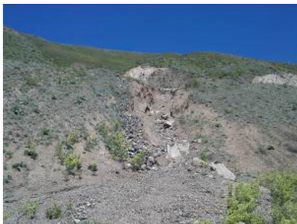
Slope Collapse from Road Shoulder to Lower (DEP30) Slope Collapse on Cut Slope (BNT Road)
