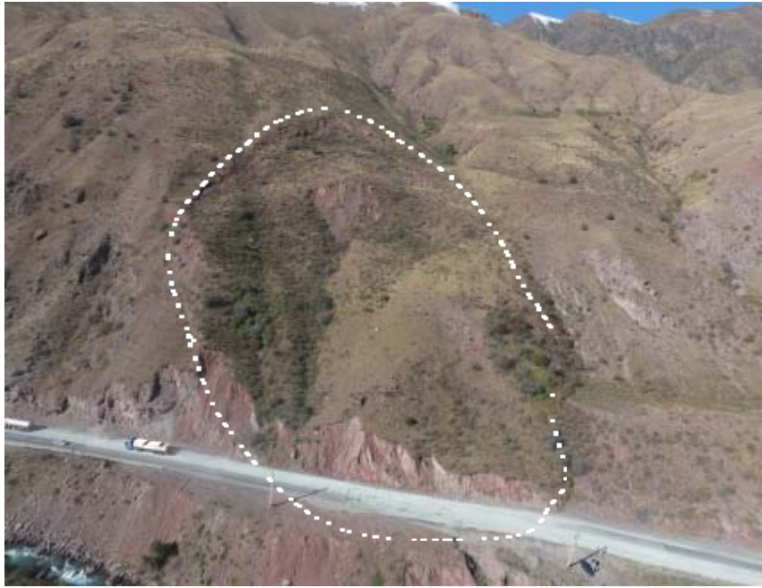
Photo 2.1-3 Deformed roadway due to landslide (DEP9)
