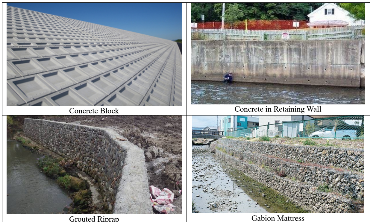
Figure 7.2-2 Sample of Revetment Type
