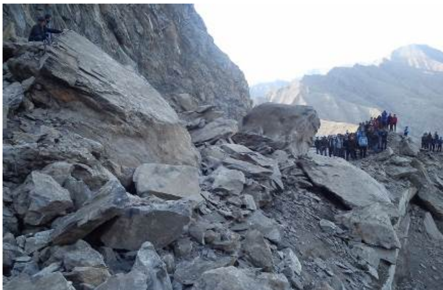
Photo 2.1-1 Blocked Vehicular Traffic due to Rockfall (DEP30)
