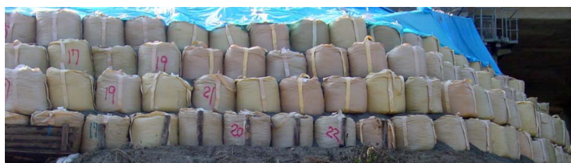
Figure 10.3-16 Banked up large sandbags
