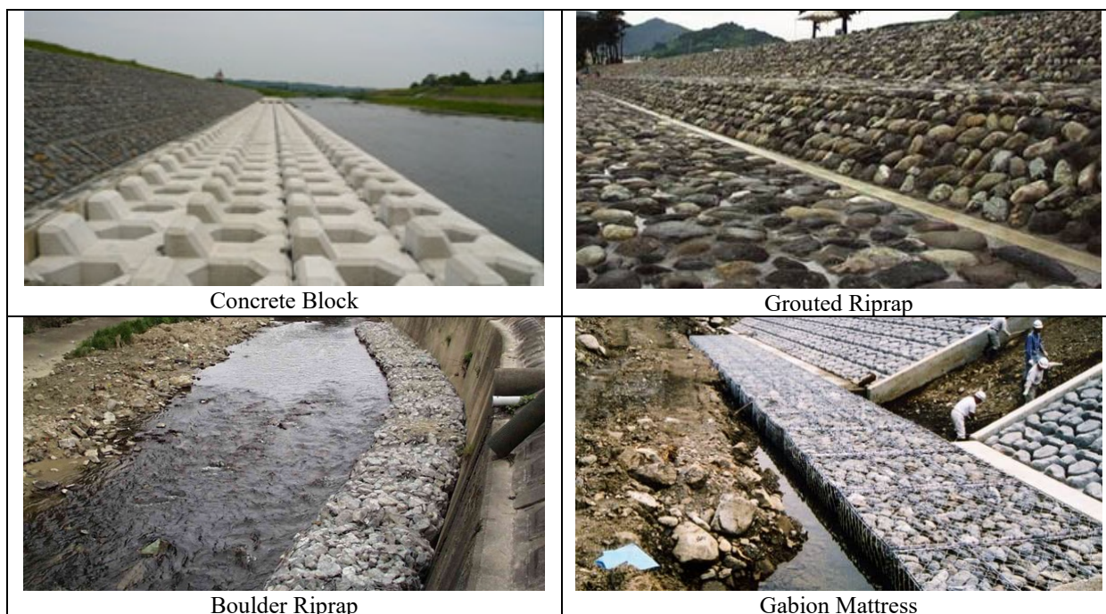
Figure 7.2-3 Sample of Foot Protection Type
