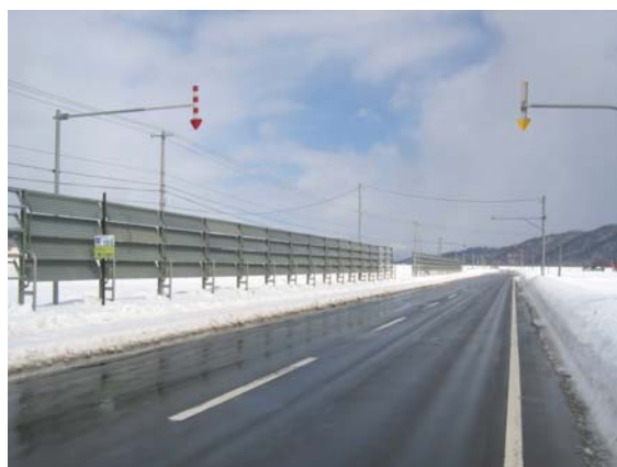
Photo 9.3-5 Blower Snow Fence
