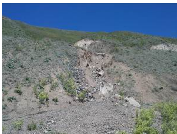
Slope Collapse from Road Shoulder to Lower (DEU-30)
