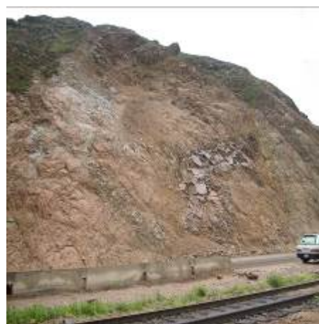
Slope Collapse on Cut Slope (BNT Road)
