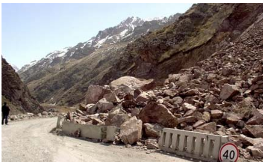
Accumulated Rocks at Back of Wall (DEU-9)
