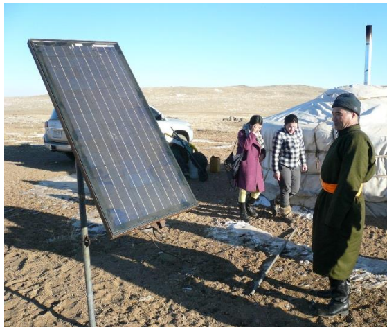
A solar panel installed near a ger
