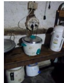
Photo 7: Electric Appliances (Rice cookers and a water boiler)
