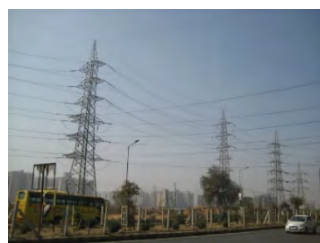
Transmission Lines (Gurgaon)
