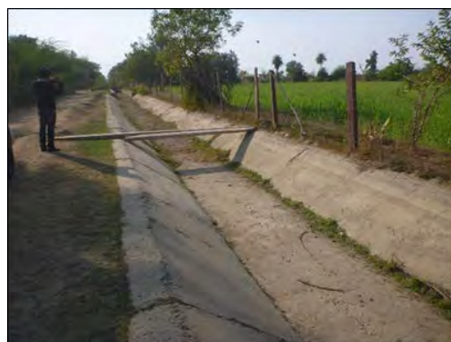
Cleaned canal (section improved by this Project)
