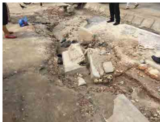
Photo 4. Collapsed Side Ditch and Side Walk Due to Heavy Rain
