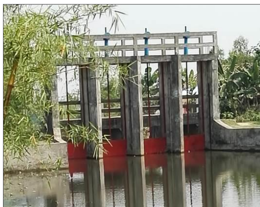
Constructed sluice gate (Binna Kandi SP : Sylhet)
