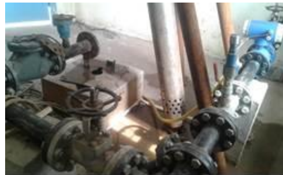
Photo 4. Intake facility of new tube well not used due to breakdown (Dobathar No. 3)
