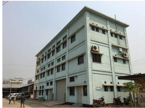
Photo 4: Building for storeroom and training of DNCC
