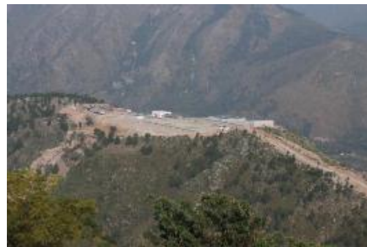
Photo 1. Newly constructed water treatment plant of the surface water supply system (a distant view as of July 2015)
