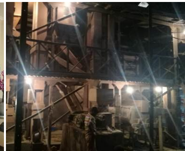
Milling factory where electricity is indispensable (Sylhet)
