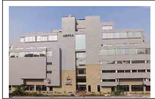
National Electric Power Regulatory Authority (NEPRA)
